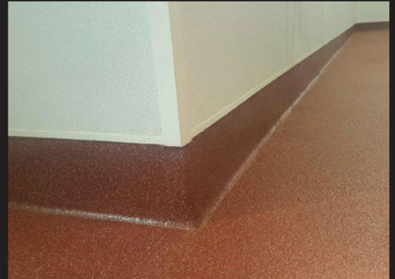
Integral 4" or 6" cove base creates a bathtub effect for effective waterproofing.
